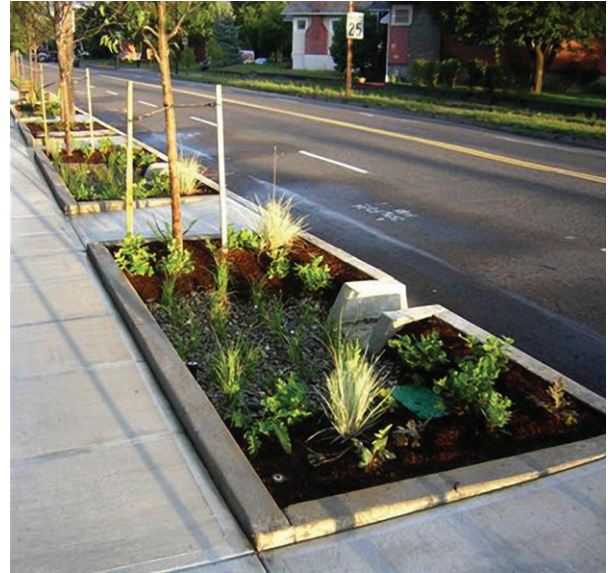
BMPs such as vegetated swales and tree well infiltration pits offer stormwater capture benefits as well as pollutant reduction and groundwater recharge benefits.
