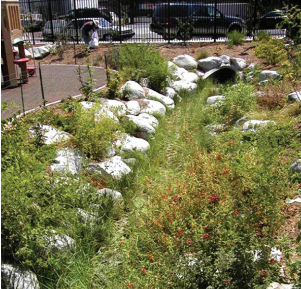
BMPs such as vegetated swales and tree well infiltration pits offer stormwater capture benefits as well as pollutant reduction and groundwater recharge benefits.
